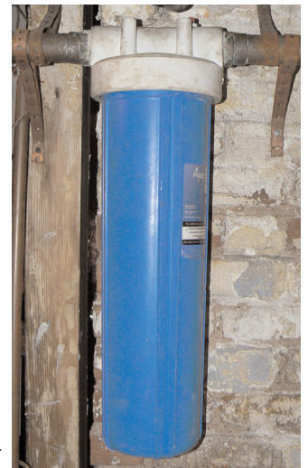
A 20 INCH 'BIG BLUE' FILTER HOUSING
